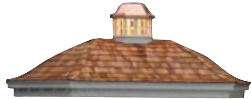
Cedar Shake Roof
